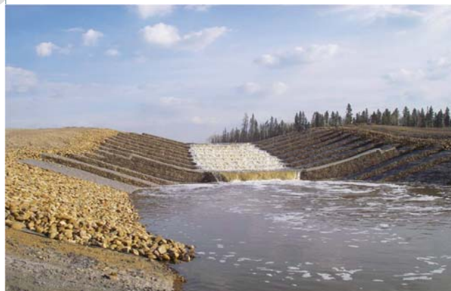
Figure 3: Reno ® mattress Castoro Polimac coated
